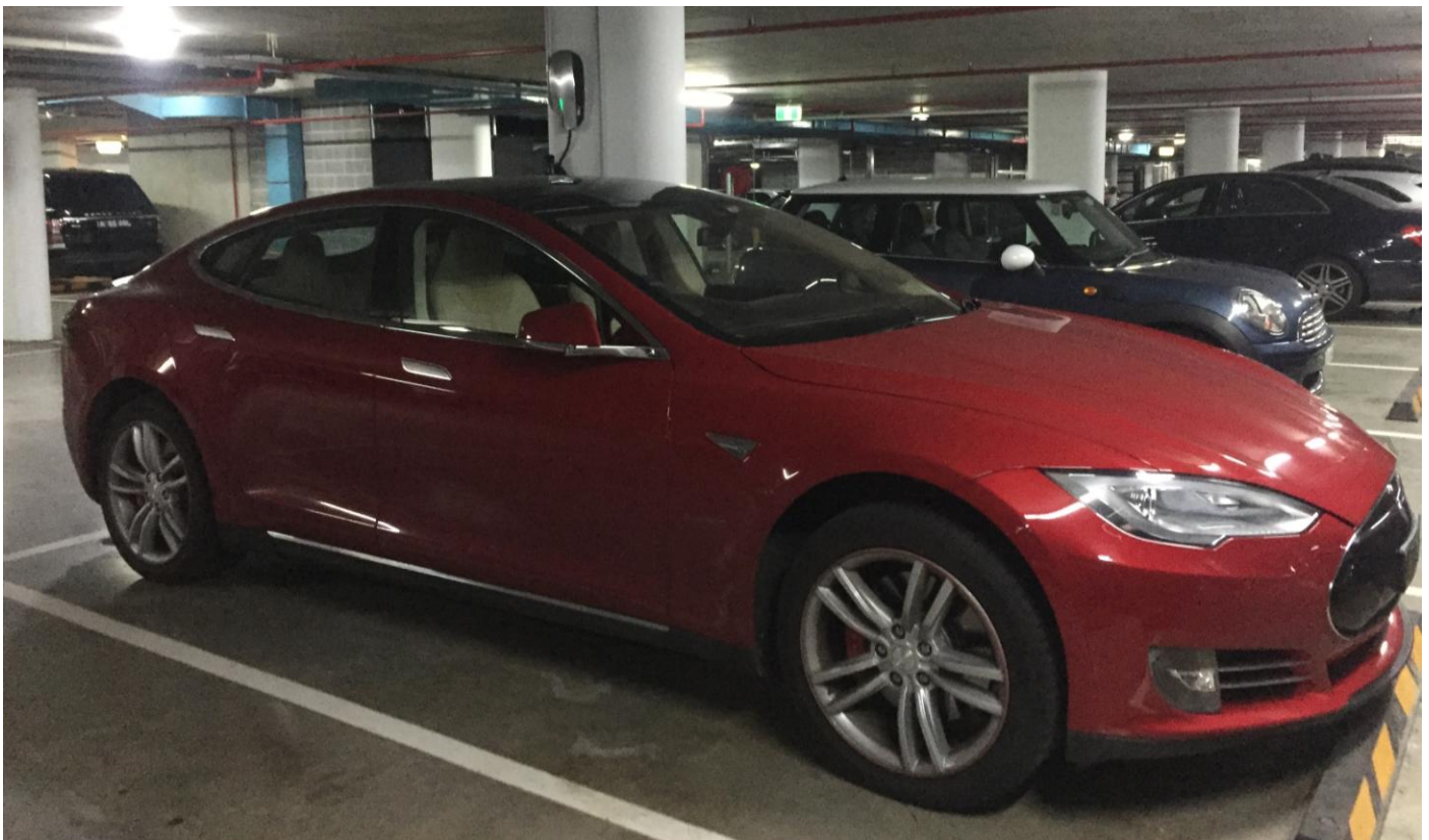
Figure 25: Electric Vehicle with dedicated charging unit installed
