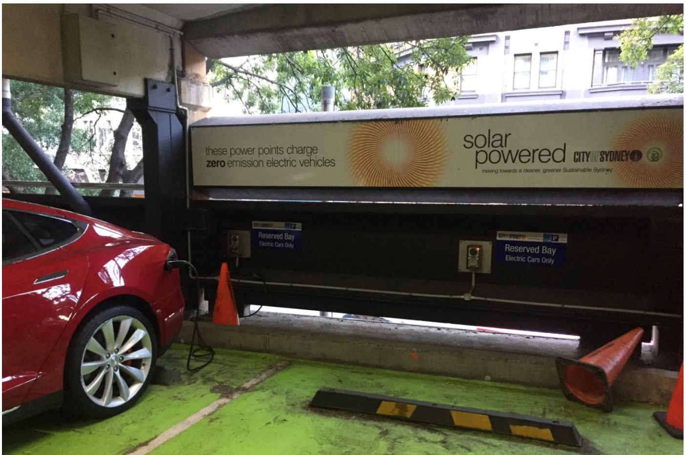
Figure 50: Goulburn Street Car Park
