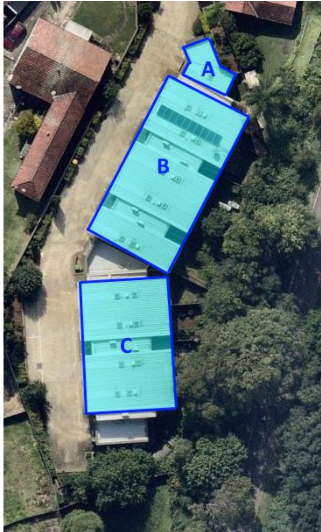
Figure 4: Orientation and tilt zones on the roof of 6 Noel Avenue, Adamstown
