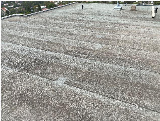
Figure 32: The waterproofing on the rooftop of the building – not conducive to Solar Panel installation
