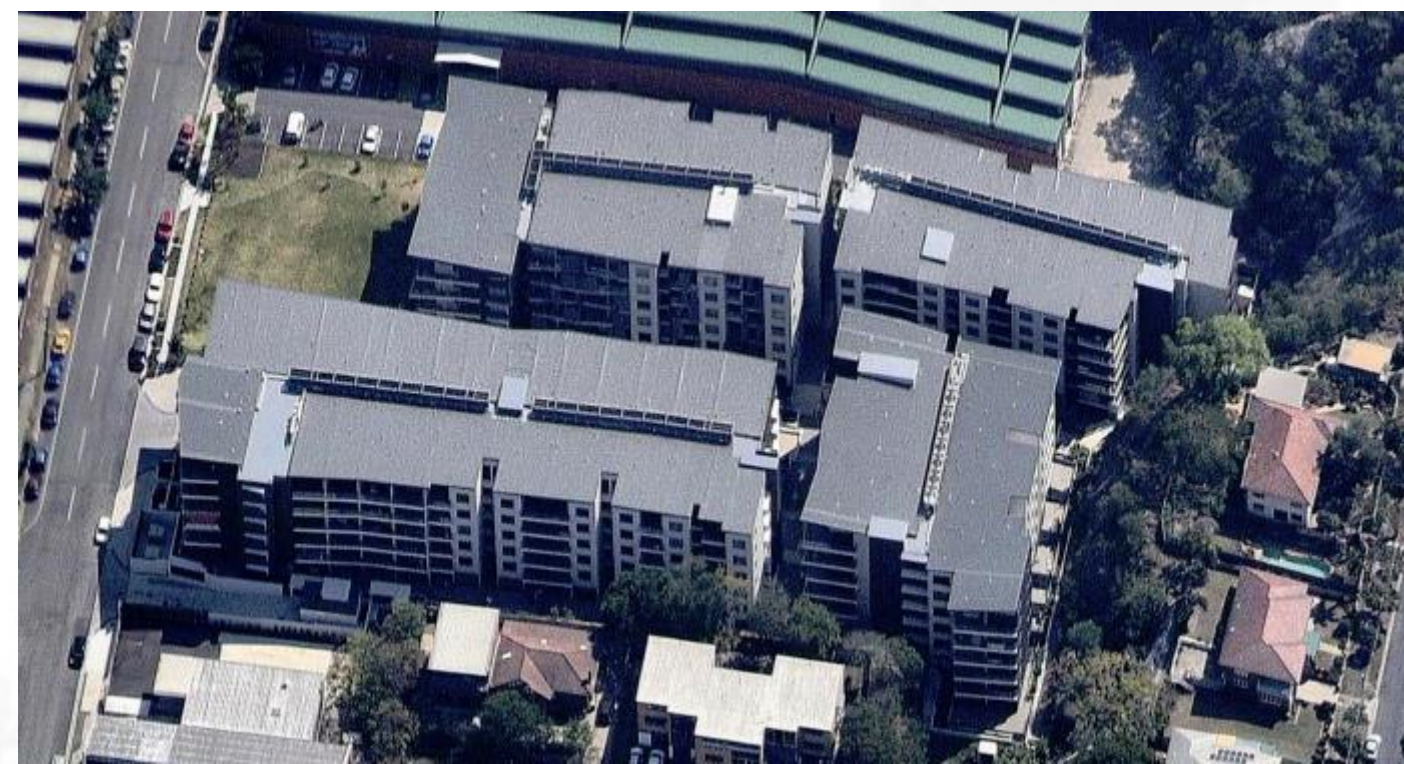
Aerial view of Jade
