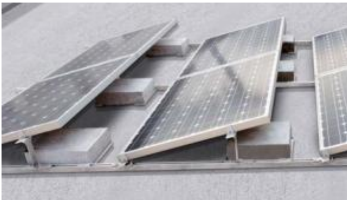
Figure 10: Ballast mount solar system (Roofing Contractor, 2014)
