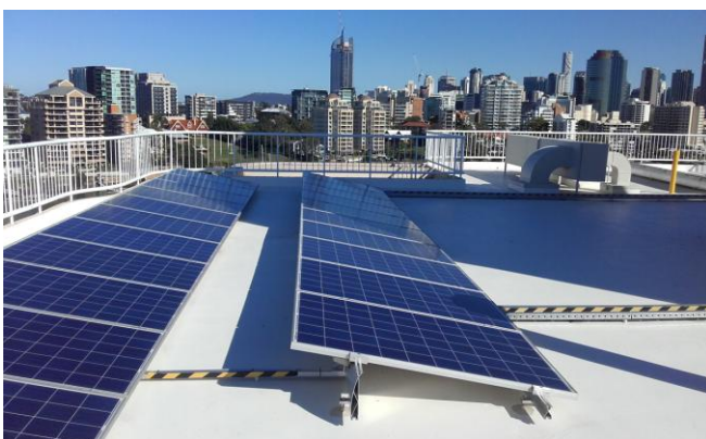
Figure 9: Flash mount solar system (Roofing Contractor, 2014)
