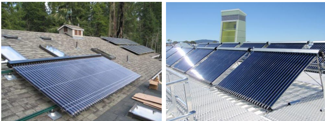
Figure 28: Examples of solar thermal hot water systems (Enviro Friendly World, 2015)
