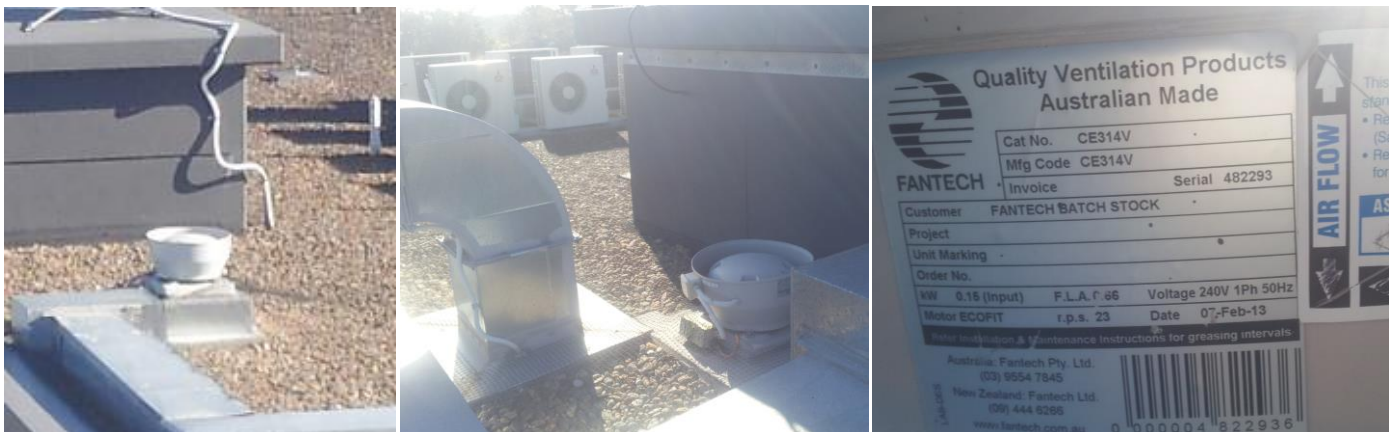
Fig. 11 From left to right, Comms topper fan Building A, Comms topper fan Building B, Rating label close up
