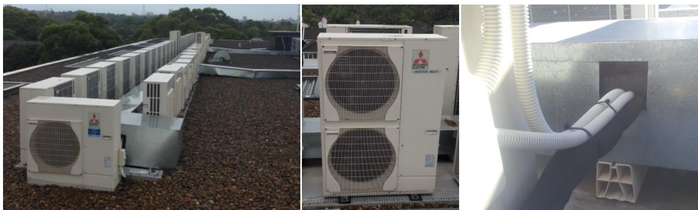
Fig. 14 From left to right, air conditioners in rows on the roof, larger units, and ductwork usage for cables and pipes
