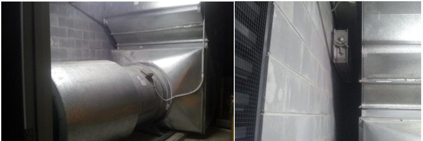
Fig. 6 From left to right, ~5.5kW Fantech exhaust fan, Carpark ductwork connects in behind the fan
