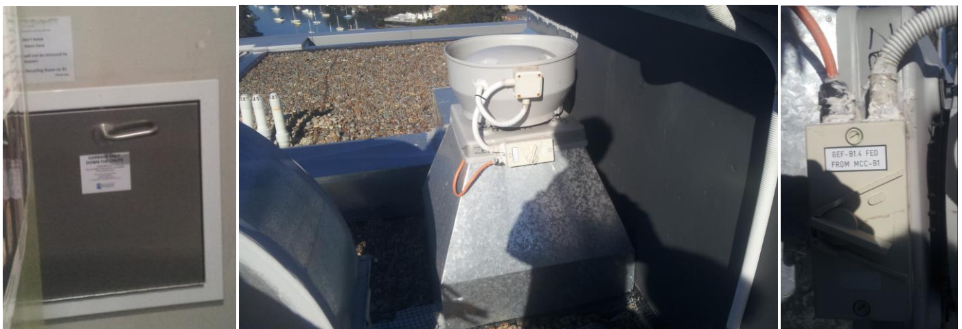
Fig. 10 From left to right, Vertical garbage shoot access on levels, with rooftop fan at the top, Control switch close up
