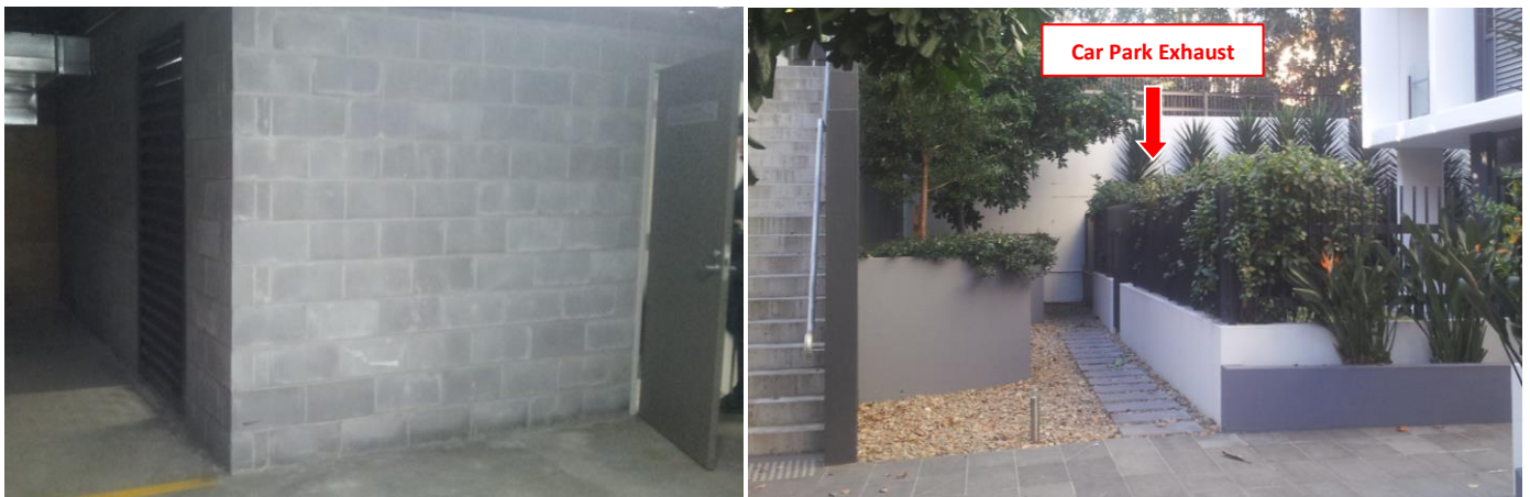
Fig. 5 From left to right, Car park ventilation room with louvered wall panel intake, External vent located in garden
