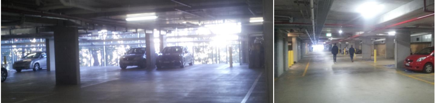
Fig. 4 From left to right, Natural car park ventilation open to the south, Length of upper car park level to entrance
