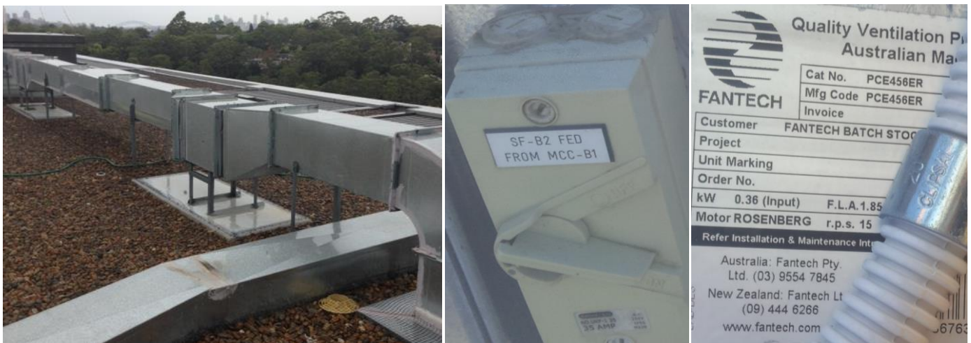
Fig. 12 From left to right, Foyer ducting on roof connects vertical shafts, Fan control switch, Rating label close up
