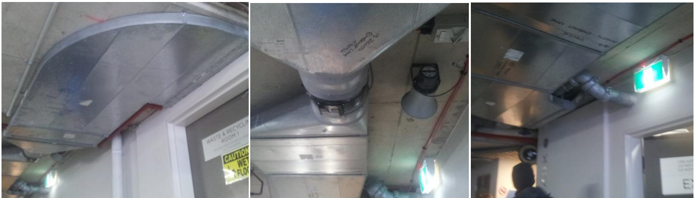
Fig. 9 From left to right, Flat ductwork from one garbage room, with in-line fan, pushes air to next garbage room
