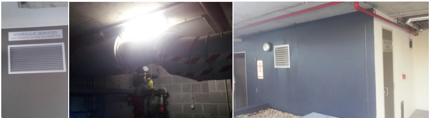
Fig. 8 From left to right, intake vent on access door, in-line fan, and vent on external wall near car park entrance
