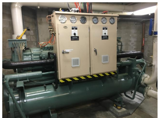
Figure 6 Chillers located in the plant room on the ground floor
