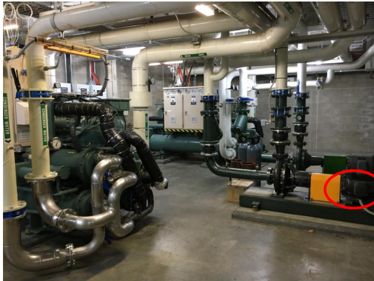
Figure 9 TECO water pump in plant room on ground floor
