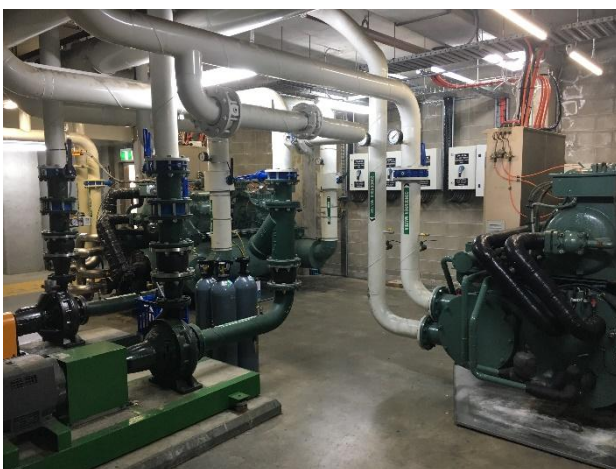
Figure 6 Chillers located in the plant room on the ground floor
