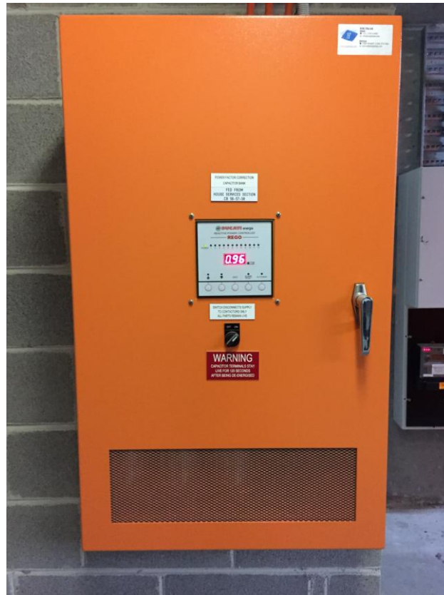
Figure 4 A 250 kVAR power factor correction unit
